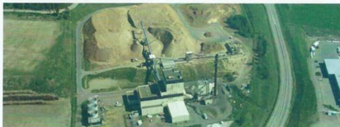
Williams Lake Power Plant
