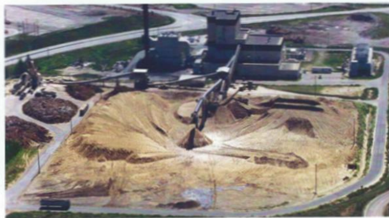
Williams Lake Power Plant
