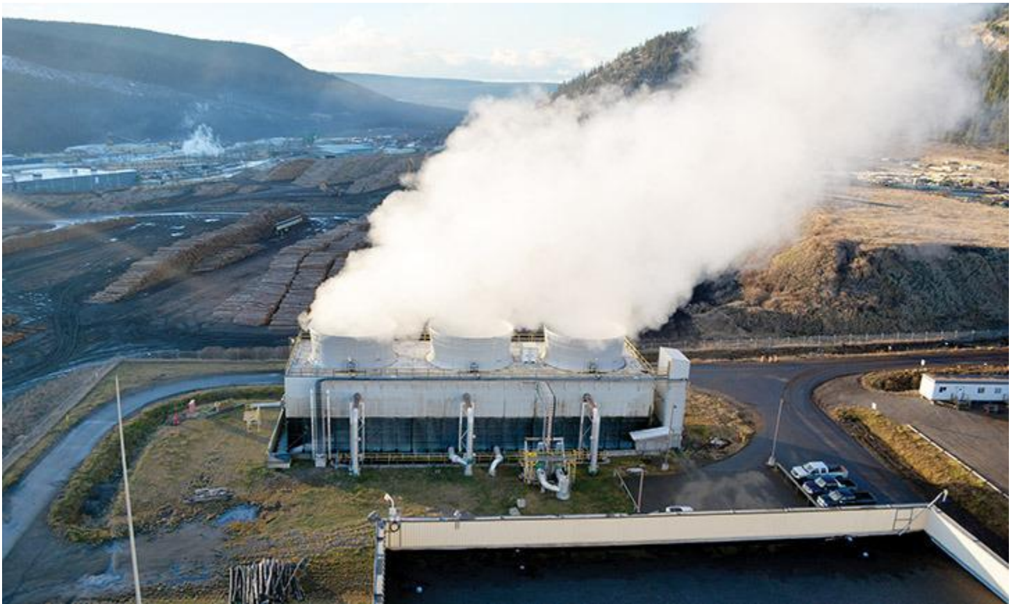
An aerial view from the rooftop of the power plant looking down on the water cooling system. — Image Credit: Monica Lamb-Yorski Photo
